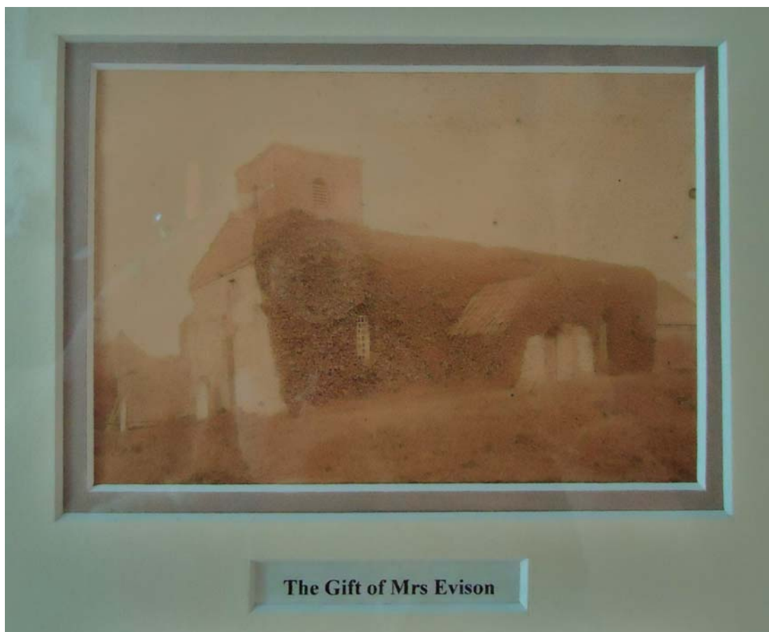
Reighton church with its old tower and porch
